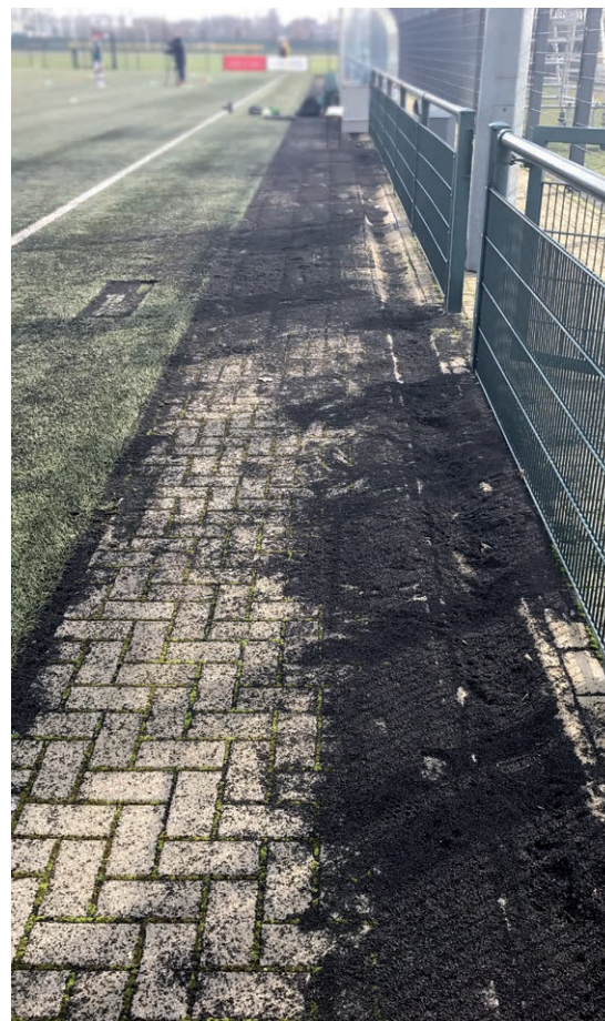
Fig. 9_Granules discharged by snow removal
