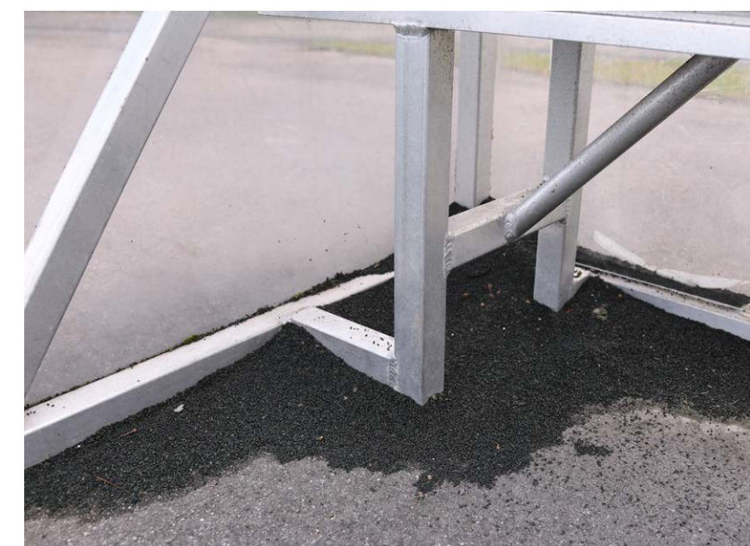
Fig. 8_Dispersed granulate under the subs' bench
